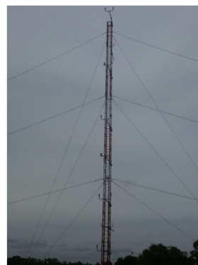
Figure 20: 32 m micrometeorological tower installed at TERLS.
